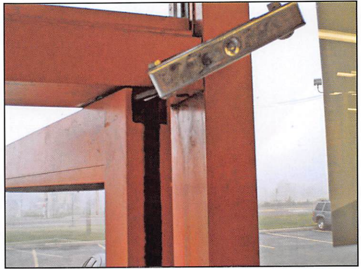
Two hex head bolts secure the door to the overhead closer. Once these are removed, the door slips off the bottom pivot and can be dropped.
