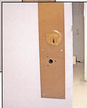
The cylinder is installed through the push plate in photo 7.
