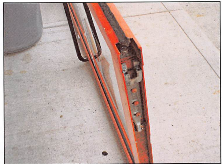
Once the door is down, we can see the arm for the concealed closer, as well as how it attaches to the pivot of the concealed closer.
