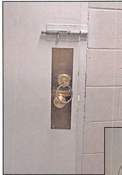
Photos 8 and 9 show the finished install. The customer was advised to remove the barrel bolt that was installed as a temporary fix.
