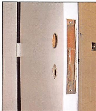
The mortise pocket and existing holes are seen photo 2.
