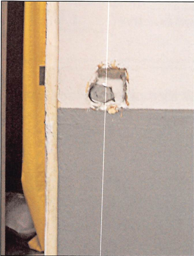
Photo 10 shows the old inside spindle hole. The padding on the cell door has been scratched away with fingernails over the years. A patch made with the DonJo hole filler can be seen in the lower left corner of the hole.
